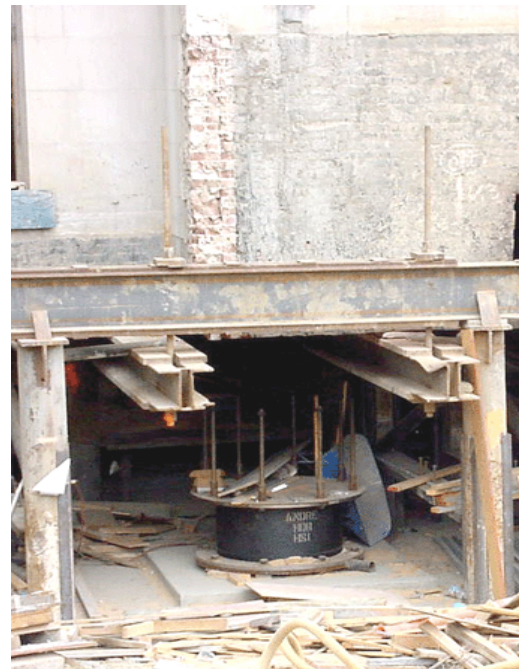
Fig. 1.3: The left panel shows in a sketch how seismic base isolation works. A base isolator mechanically separates a building from its foundation anchored in the ground. When the ground vibrates in an earthquake, the rubber and steel laminate absorbs much of the movement and prevents the building from shaking. The right panel shows a base isolator underneath the raised Hearst Memorial Mining Building during its installation in 2000.
