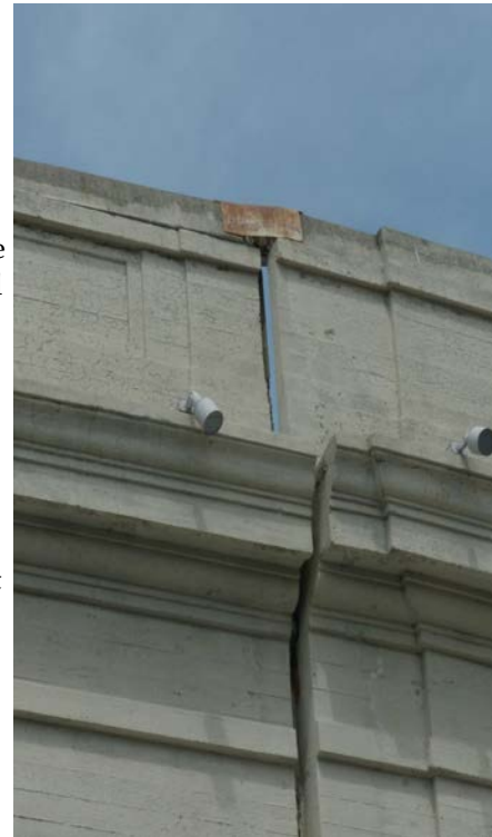
Fig. 5.10: The famous gap in the exterior wall at section KK as seen from outside the stadium in April 2017. Note the rusty metal cap, a relic from long before the reconstruction of the stadium.
