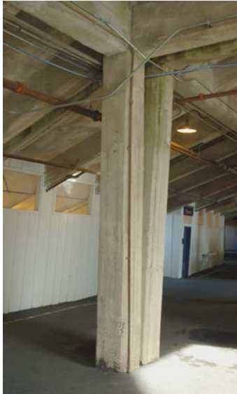
Fig. 5.12: This picture was taken on the concourse level below section KK in December 2008. It shows typical support columns before reconstruction. Due to fault creep the two neighboring columns are tilted with respect to each other and hence misaligned. Note that the water and electric lines are fixed and not flexible.
