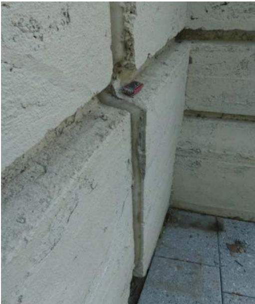
Fig. 5.7: Here two sections of the exterior stadium wall meet. The fault creep has moved the sections about 1.5 inches apart. During the renovation, the expansion joint was filled with flexible sealant.
