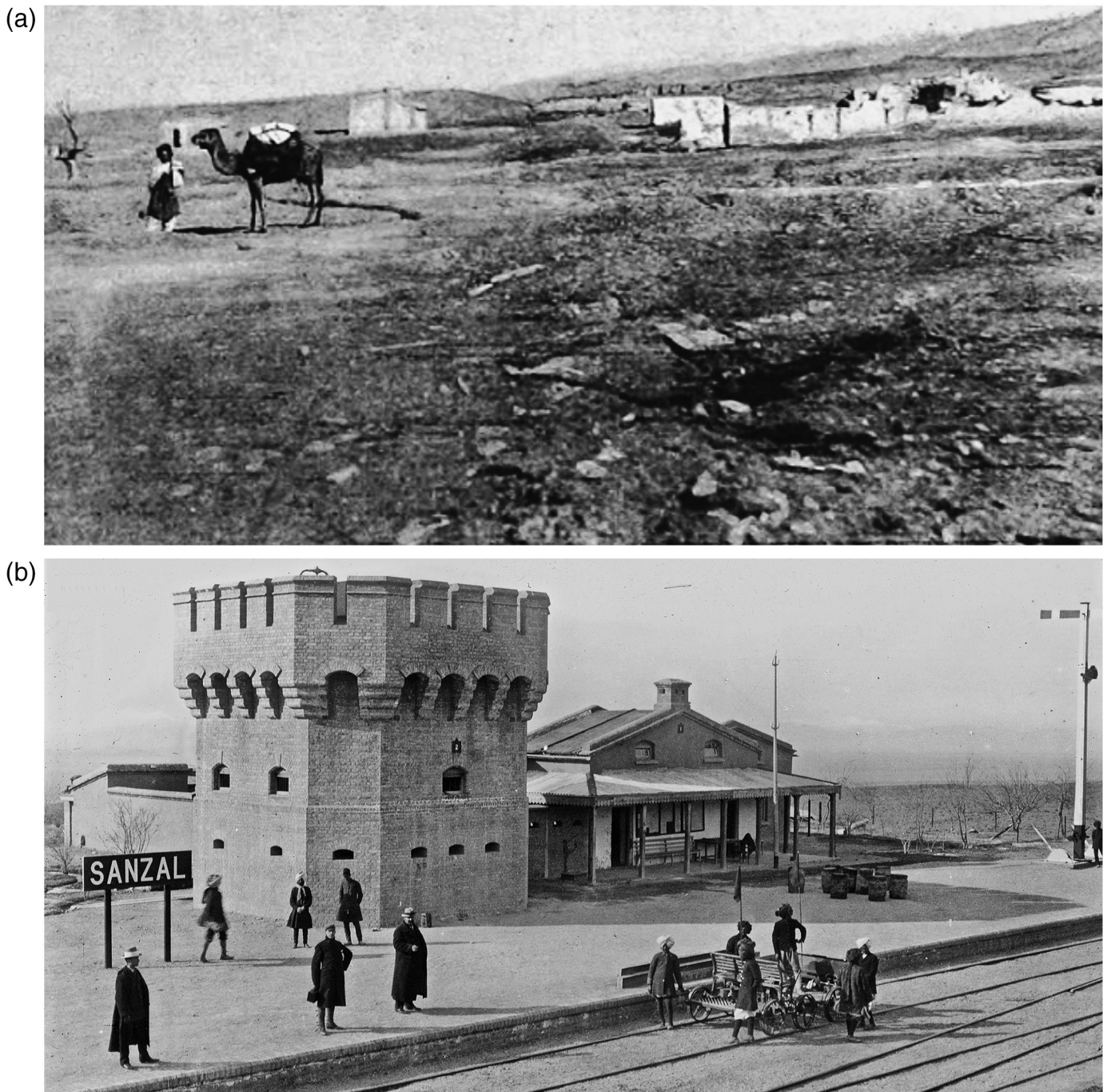
▲ Figure 2. (a) North-northeast view of the Chaman rupture of 1892 showing the mole track of the surface rupture running from the foreground to the distance between structures in Old Chaman (Egerton, 1893). Some roof collapse may have occurred to structures within 30 m of the fault (intensity 7 < EMS < 8 ). (b) View of Sanzal station (700 m from the fault) repaired 3 yr after the earthquake (Jackson, 1895). The tessellated masonry structure supports an open water tank. EMS, European Macroseismic Scale.
