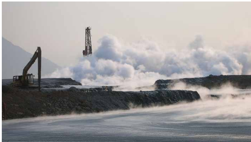
Lusi's enormous size dwarfs excavation equipment. Rising steam hovers over the volcano's vent, obscuring piles of dirt that are part of the levee system built to contain the mud.
