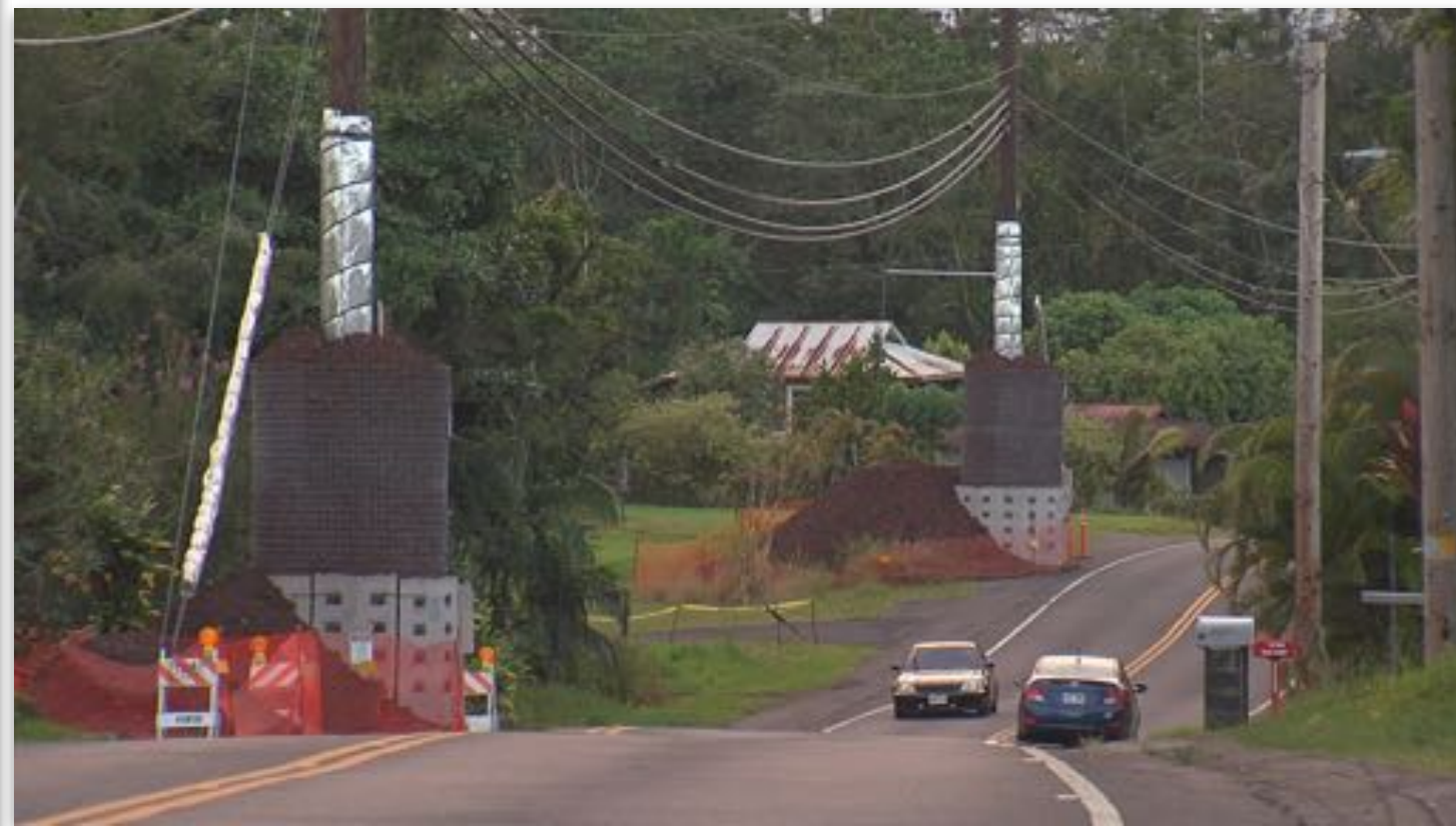
Protecting power poles in Pahoa, 2014
